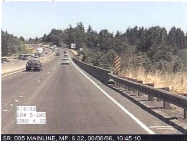
Salmon Creek Bridge (Northbound)
