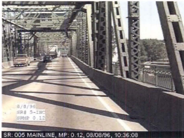
Columbia River Bridge (Northbound)
