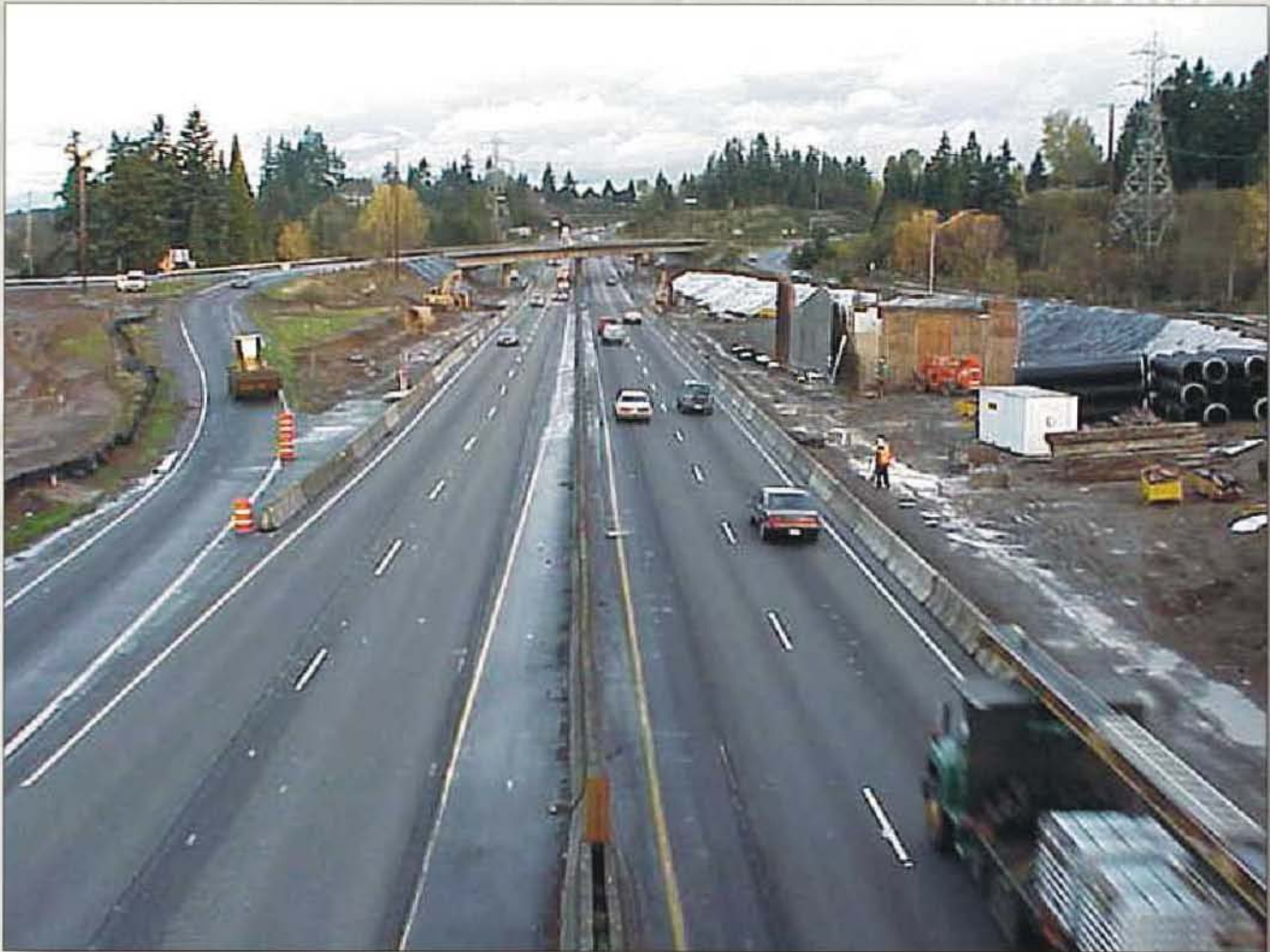
Construction on I-5 at Highway 99
