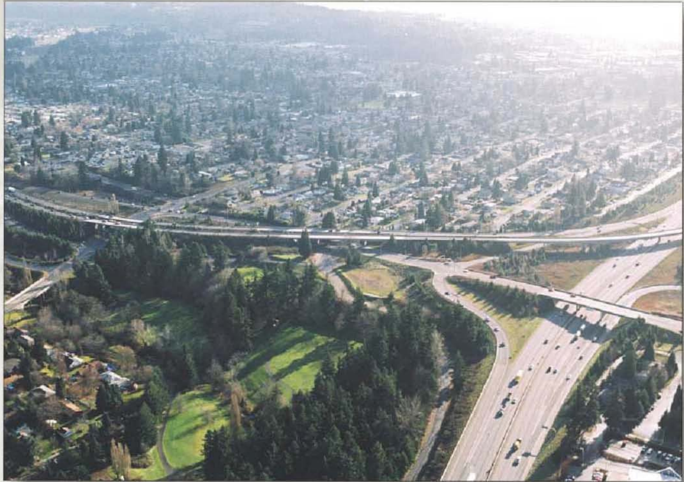
I-5 / SR 500 interchange
