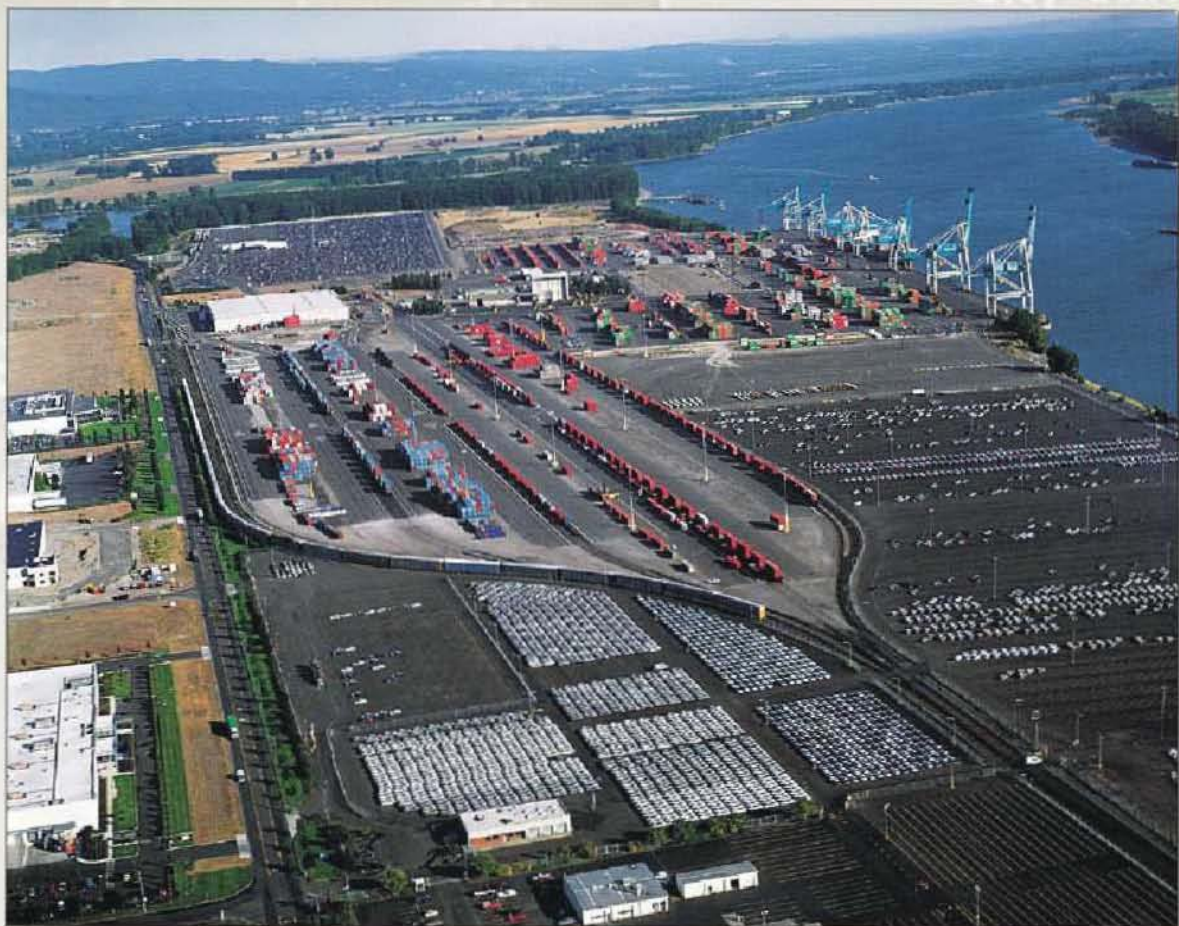
T-6 Intermodal Facility, looking west
