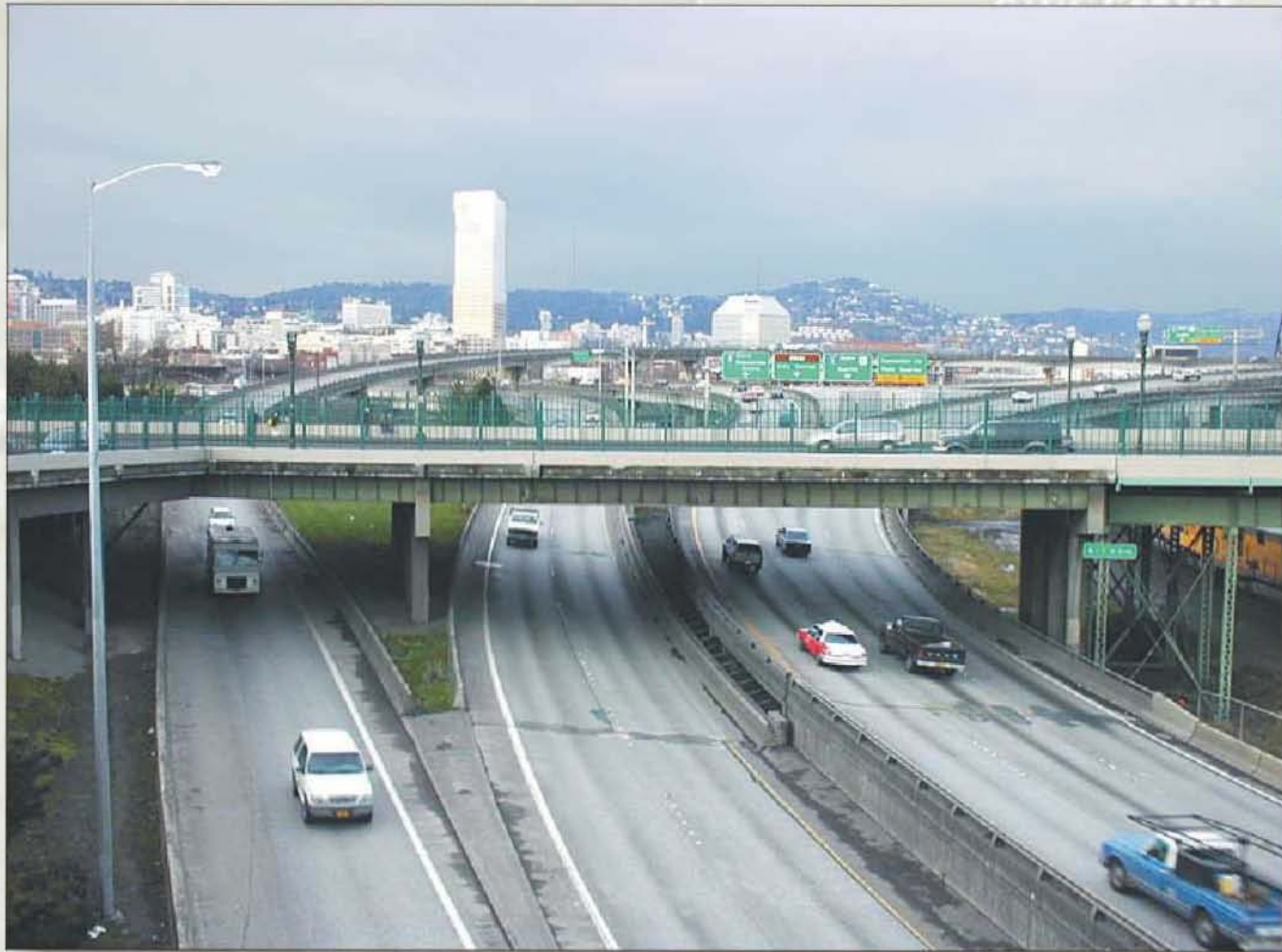
I-5 / I-84 junction, looking west
