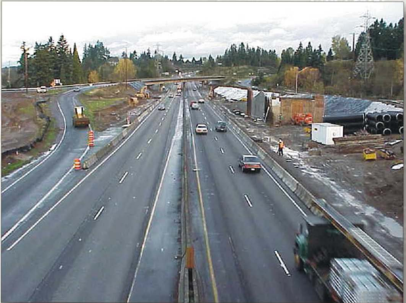
Construction on I-5 at Highway 99
