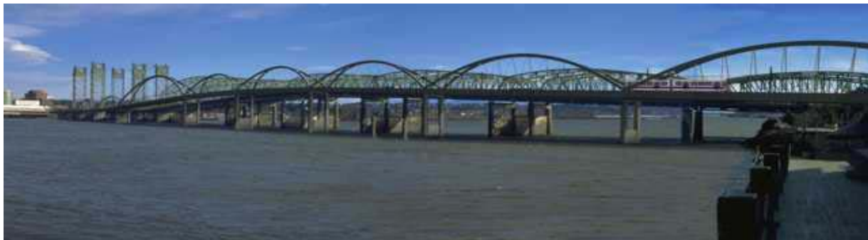
Simulated Bow Sting Arch LRT Bridge, Down Stream of the Existing I-5 Bridges (This rendering is an example. Selection of an alignment, and bridge type has not taken place.)
