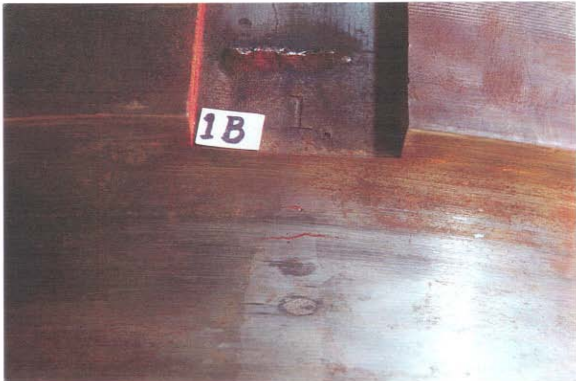
b) Defect 1B. Note dissimilar metals defining the weld filled oilway
