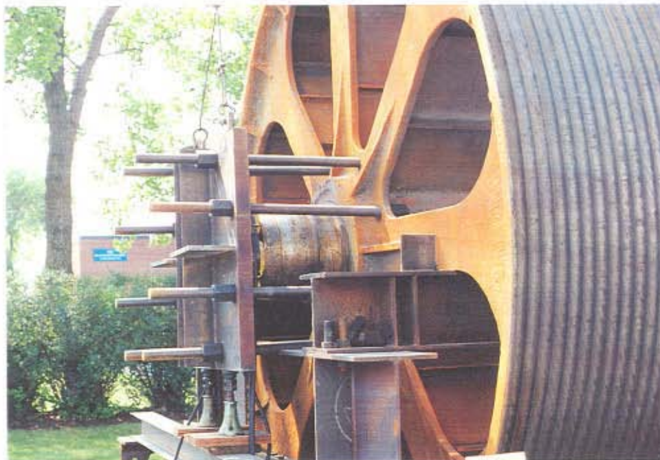
Fig. 2.4 – Jacking system used to remove trunnion intact
