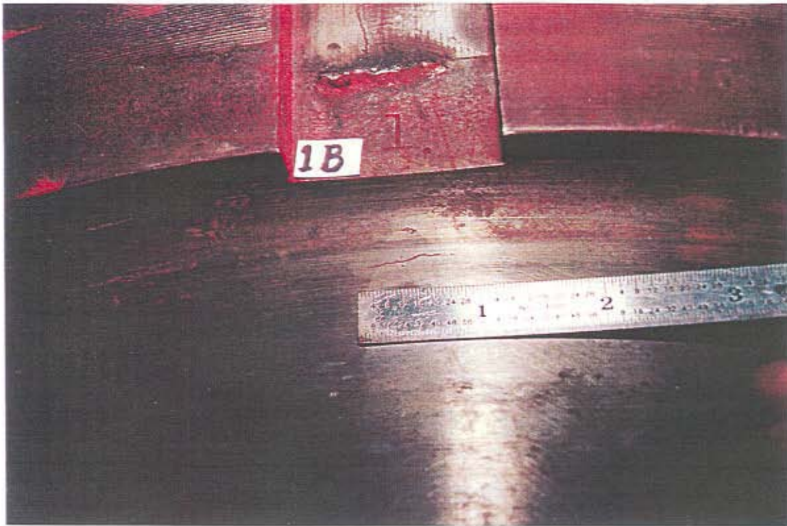
Figure 4 - Surface Discontinuity Detected by MT at Oilway Weld Repair Near Keyway 1B. (Photo Courtesy of WJE)
