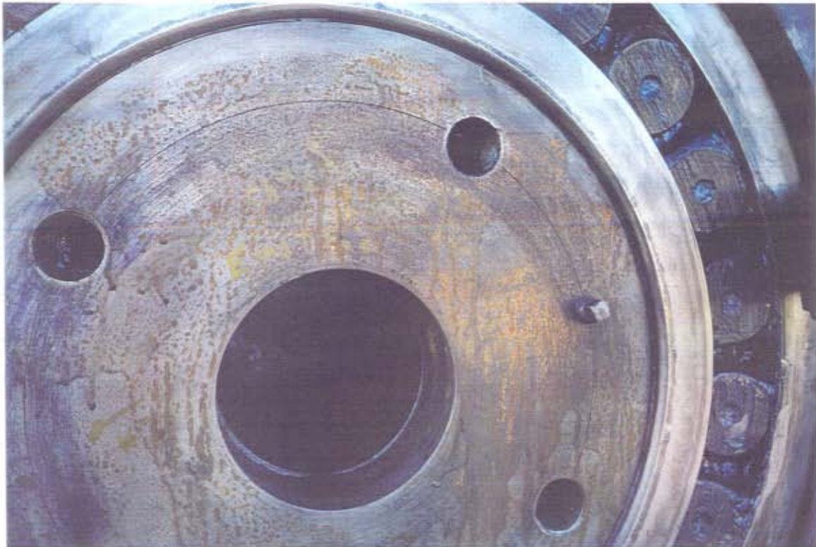
Fig. 5.1 – Preparation of south tower trunnion for ultrasonic examination
