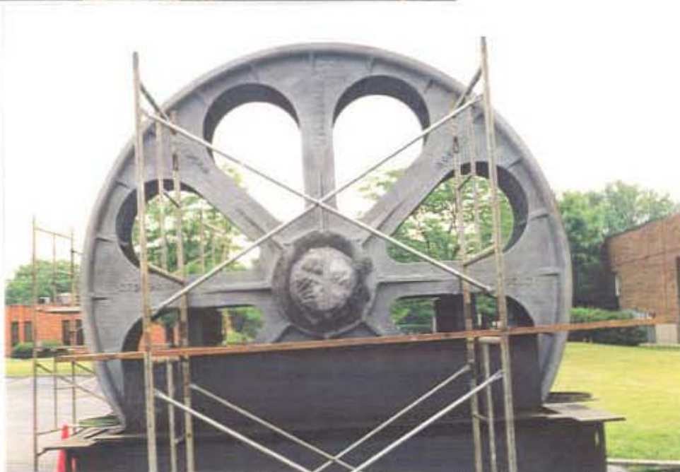
Fig. 2.2 – Sheave/trunnion assembly after sandblasting
