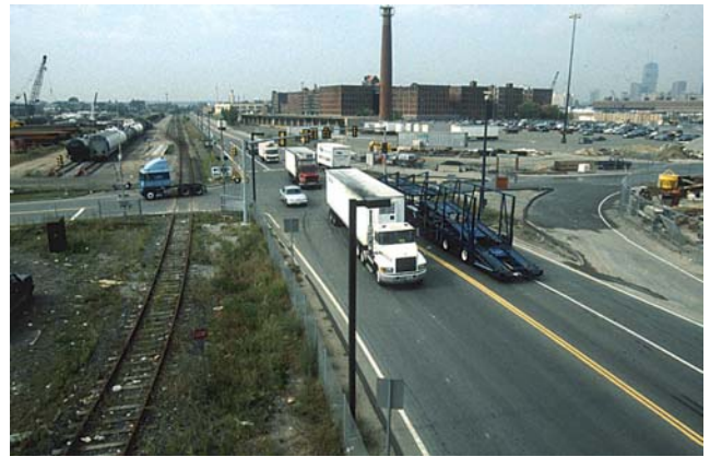
Figure 3: South Boston Bypass Road
