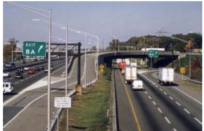
Figure 2: NJ Turnpike Dual-Dual Truck Lane
