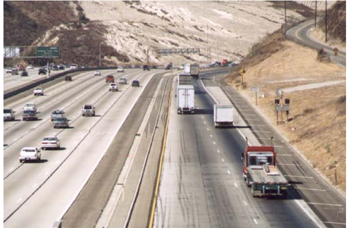
Figure 1: I-5 Truck Bypass, California (I-5/ SR-14/ I-210 Int.)
