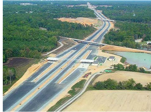
New Toll Plaza with Lanes Split for ETC and Manual Toll Collection
