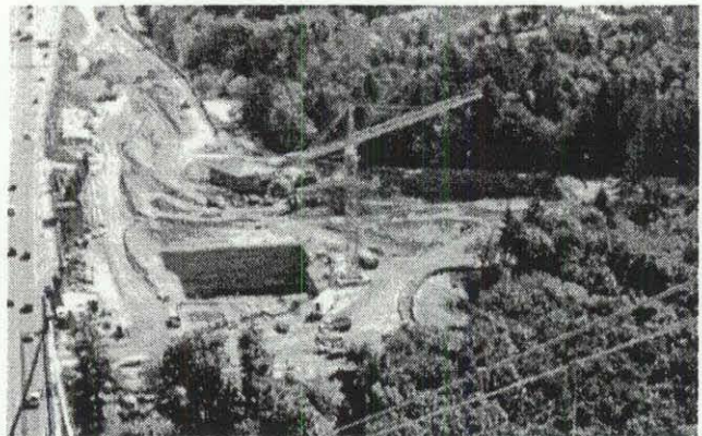
Tacoma anchorage excavation
