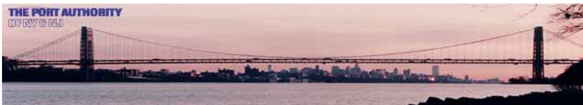
George Washington Bridge between New Jersey and New York City
