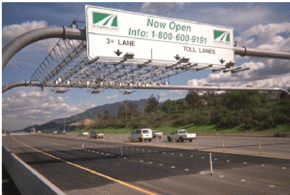
The SR-91 "Toll Plaza" is an overhead gantry HOVs use a separate lane
