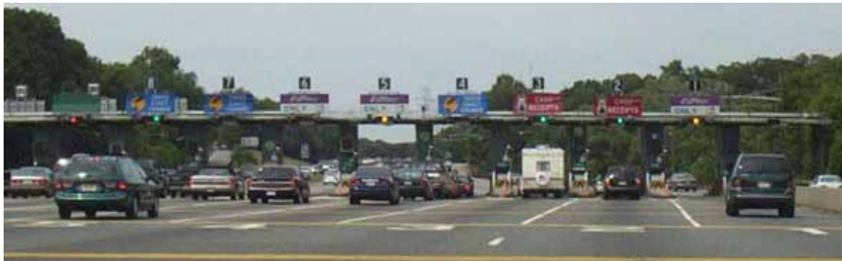
Garden State Parkway Main Line Toll Plaza
