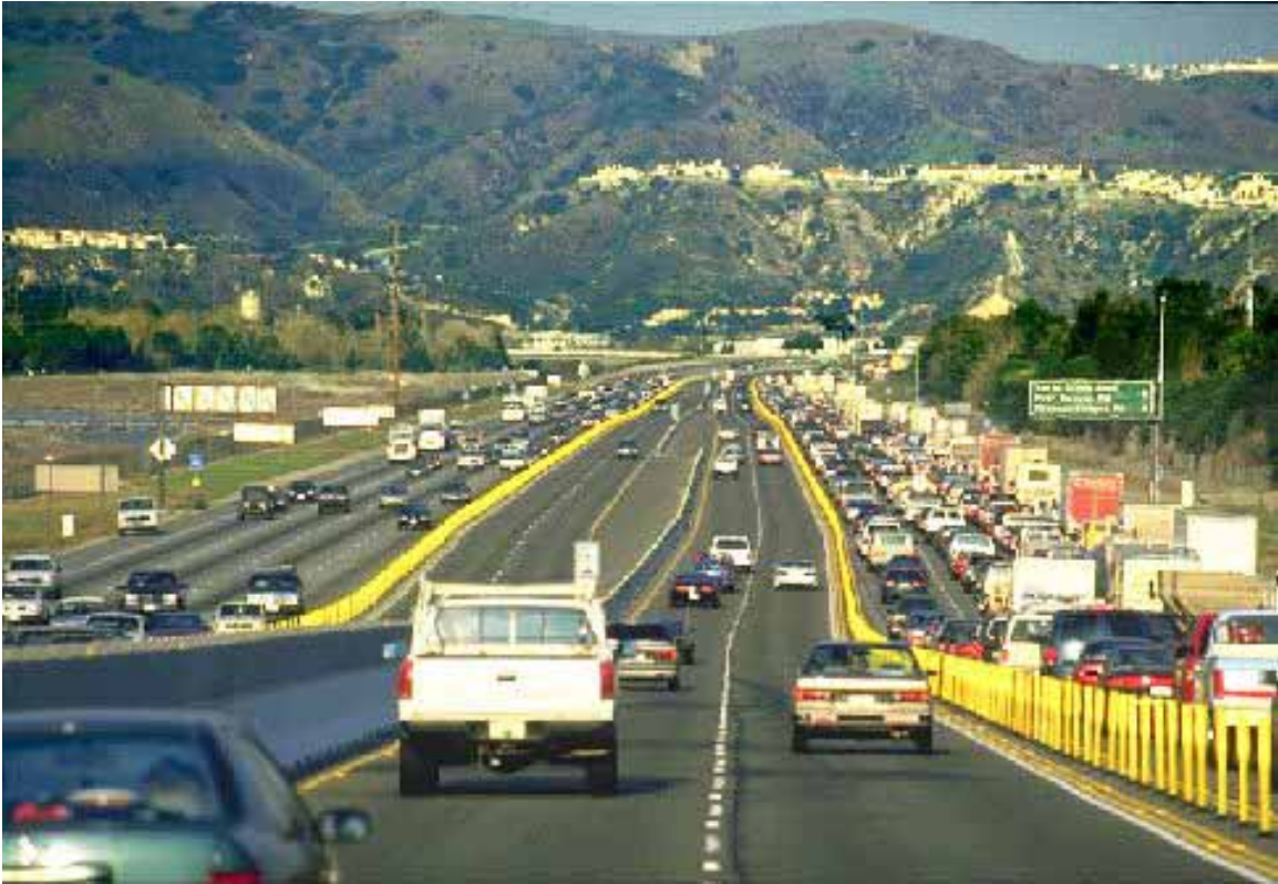
Another view of the SR-91 Express Lanes in Orange County, CA
