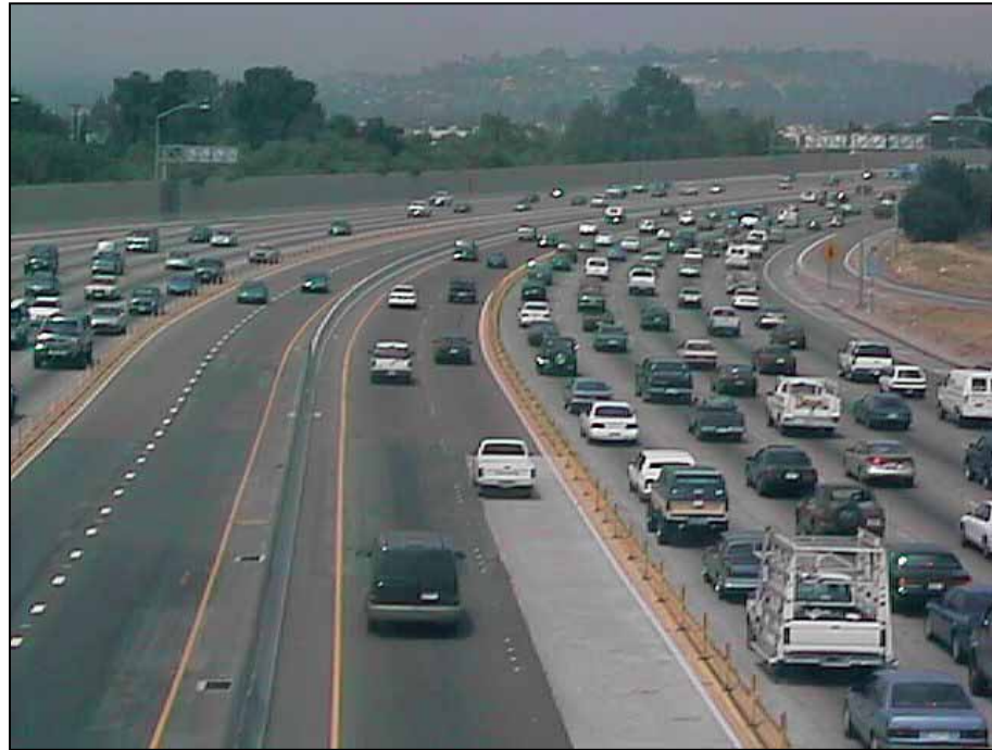
SR-91 Express Lanes – Orange County, California
