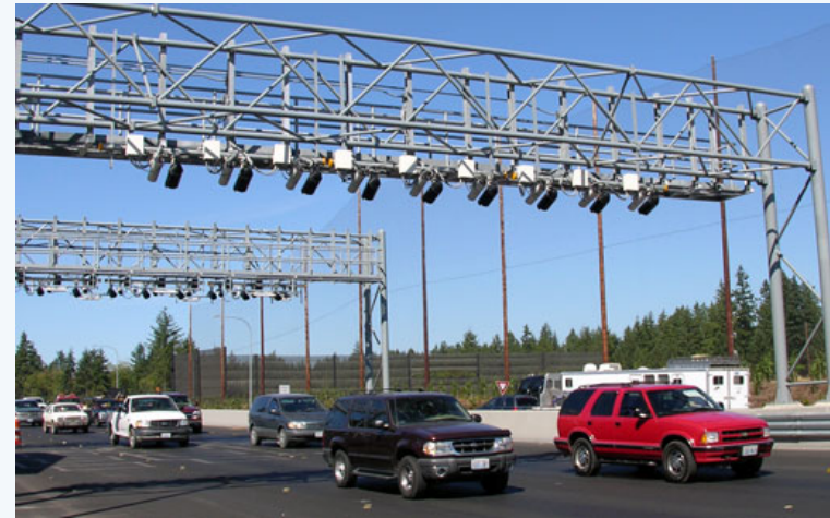
Electronic toll lanes on the Tacoma Narrows Bridge.
