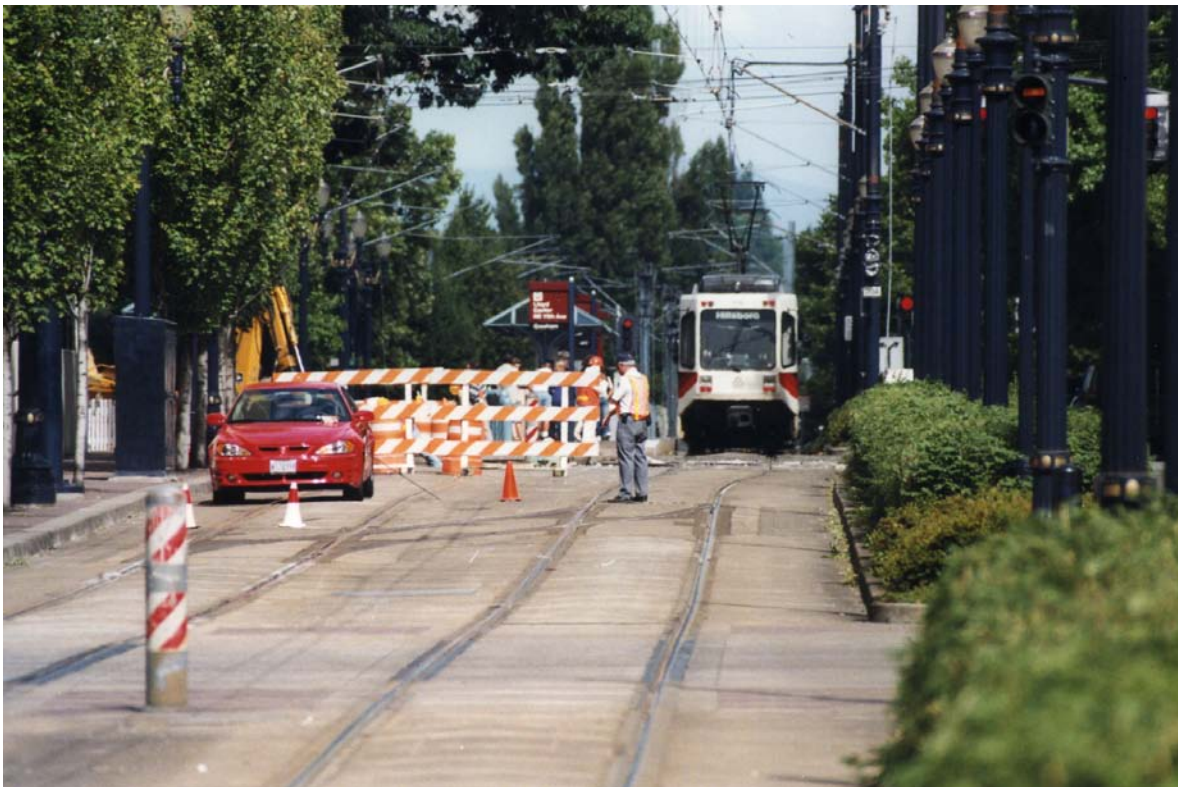
Photo: Single track operation at emergency crossover on the MAX Blue Line
