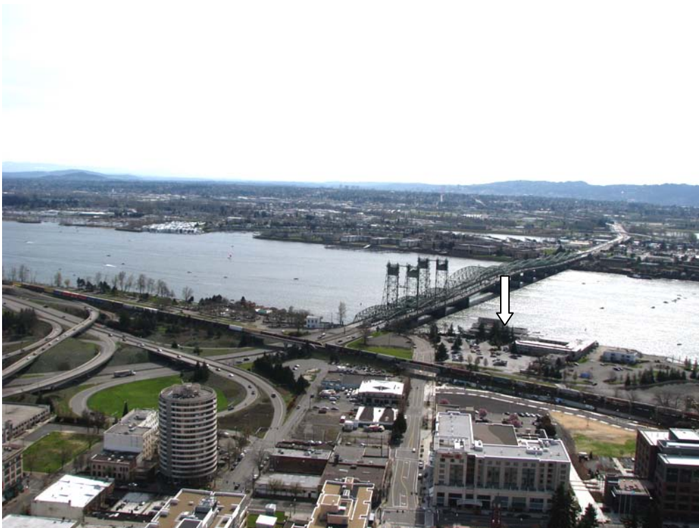
Photograph 34. Proposed Red Lion staging area on north shore of Columbia River adjacent to current I-5 bridge (03/22/08)
