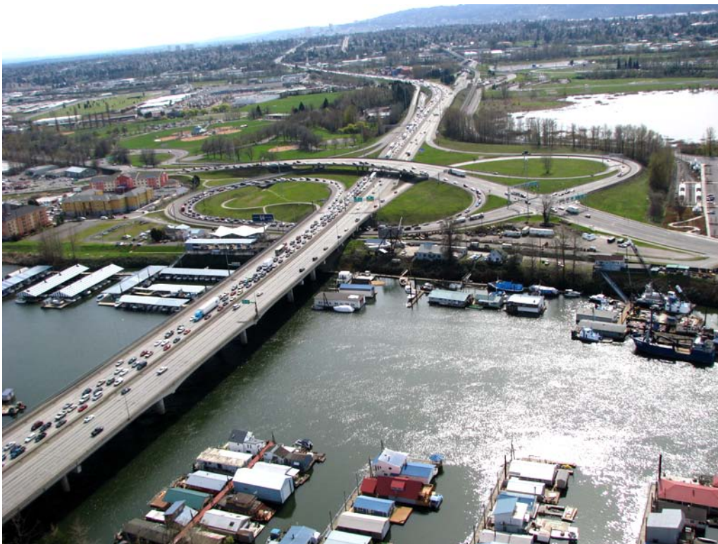
Photograph 4. I-5 North Portland Harbor bridge and shoreline looking southwest (note northbound traffic during peak hours) (03/22/08)
