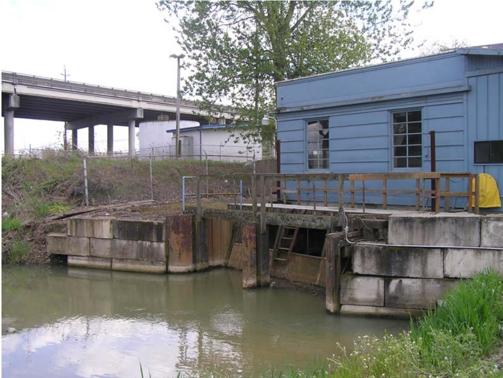
Photograph 25. Columbia Slough pump house near I-5 crossing (04/11/06)
