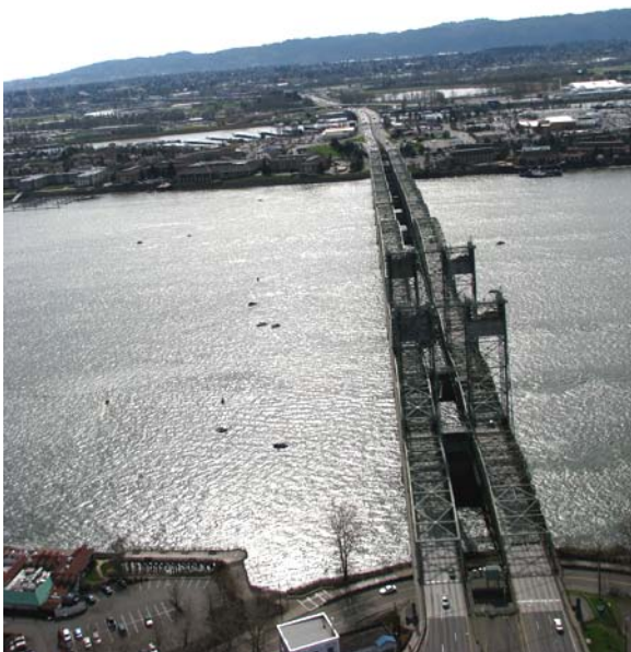
Photograph 10. Overhead view of I-5 bridges looking south (03/22/08)
