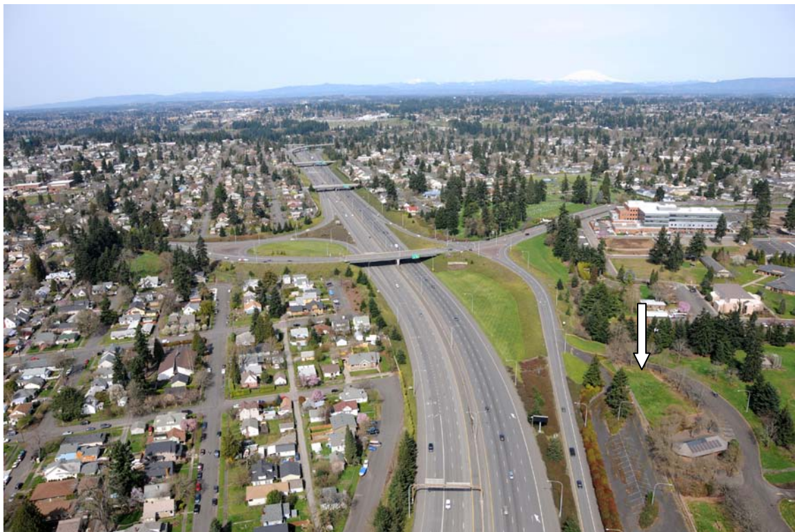
Photograph 22. Clark College park and ride proposed site in Vancouver (03/22/08)
