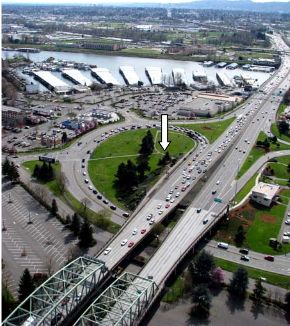
Photograph 32. Proposed constructed stormwater BMP location on Hayden Island (03/22/08)
