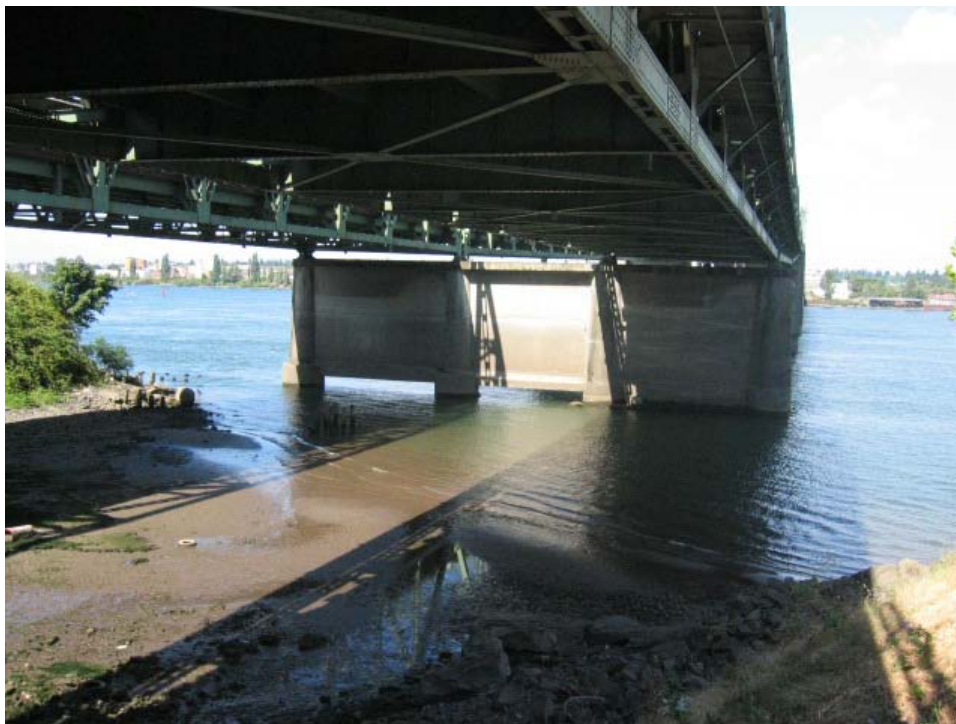
Photograph 8. I-5 bridge piers facing north from Hayden Island (08/22/05)
