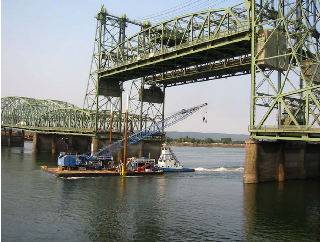
Photograph 9. I-5 Existing bridge lift towers of I-5 bridges (09/22/03)
