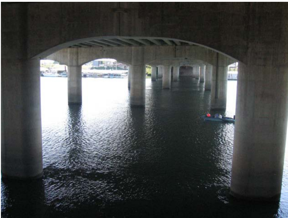
Photograph 6. I-5 North Portland Harbor bridge piers facing south from Hayden Island (08/22/05)
