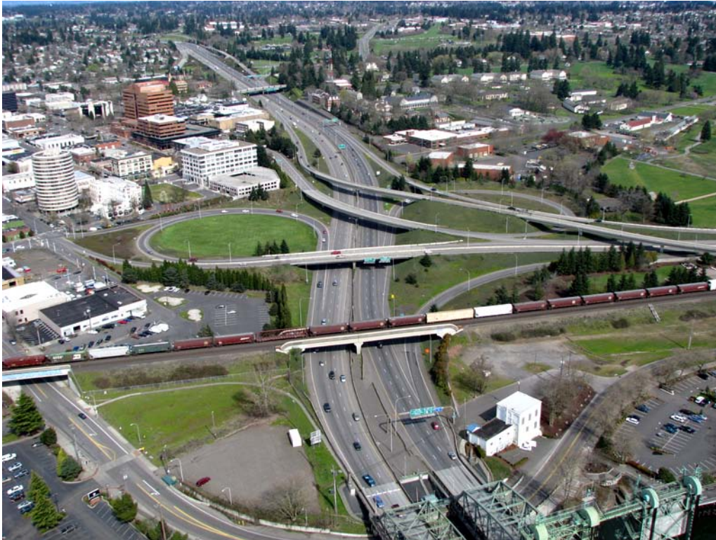
Photograph 15. Intersection of SR 14, I- 5, and BNSF Railroad looking northeast (03/22/08)
