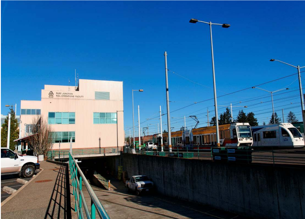
Photograph 37. Existing Ruby Junction Maintenance Facility in Gresham, Oregon (12/10/09)
