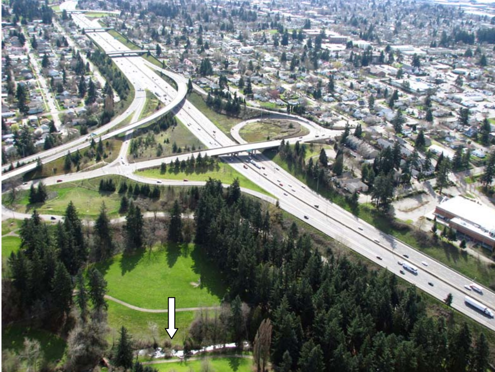
Photograph 29. Burnt Bridge Creek in the vicinity of I-5 and SR 500 (03/22/08)
