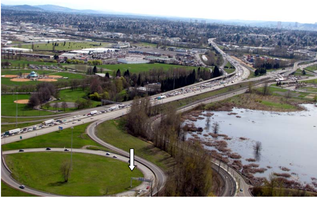
Photograph 31. Proposed constructed stormwater BMP location at Marine Drive (03/22/08)
