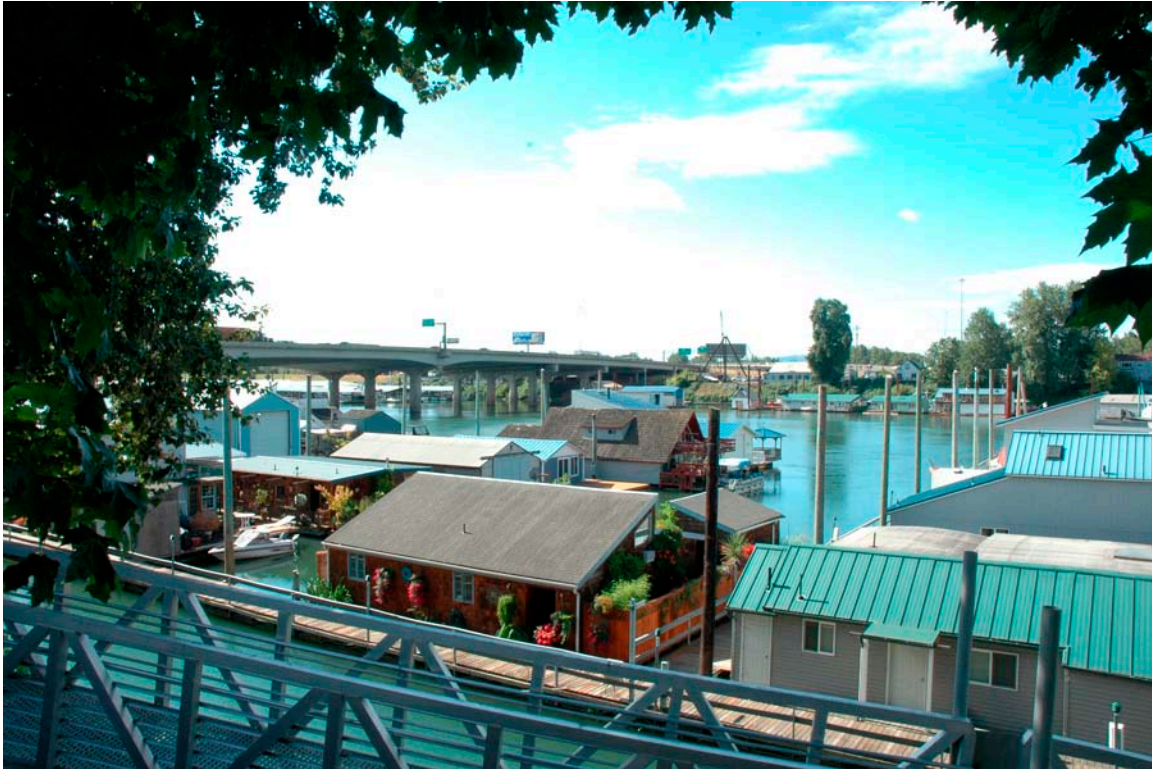
Photograph 5. I-5 North Portland Harbor bridges facing south from Hayden Island (08/16/07)
