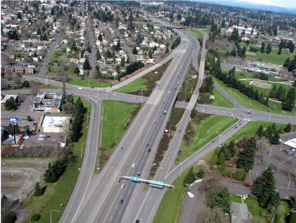
Photograph 17. Intersection of Mill Plain Boulevard and I-5 looking north (03/22/08)
