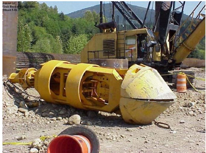
Figure 3-9. Clamshell Used for Removing Material from Drilled Shaft Casing
