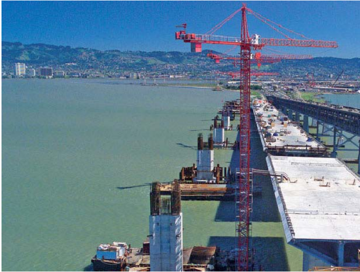
Figure 3-11. Typical Column and Superstructure Construction Using Barge-Mounted Cranes
