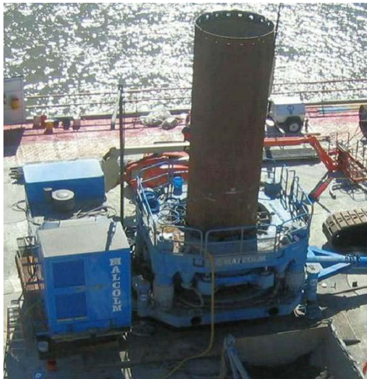
Figure 3-8. Water-Based Drilled Shaft Installation
