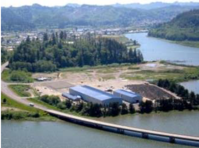
FIGURE 1-3. AMERICAN BRIDGE, REEDSPORT
