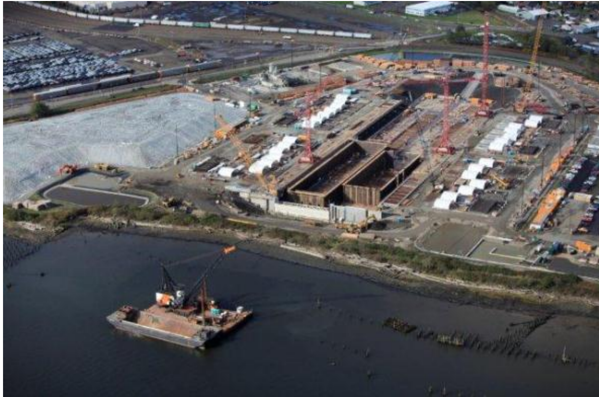
FIGURE 3-3. SR 520 PONTOON CONSTRUCTION SITE (ABERDEEN)
