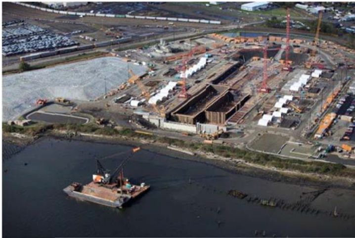
FIGURE 1-2. ABERDEEN CASTING BASIN UNDER CONSTRUCTION
