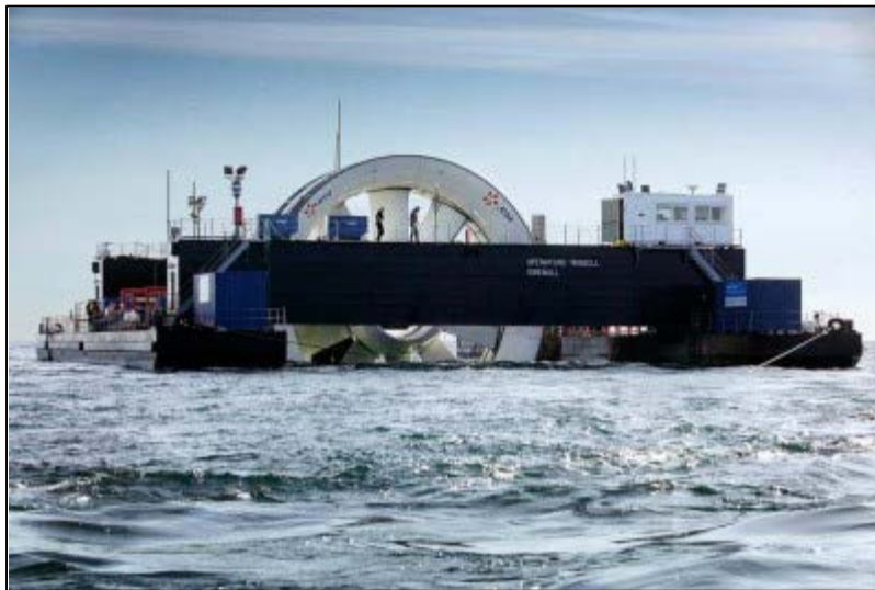
Figure 10. Deployment of an OpenHydro 2MW turbine off the coast of Brittany
