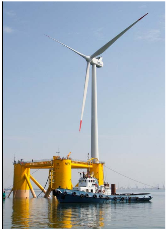
Figure 2. 2.0 MW Prototype Offshore Wind Turbine on Semi-Submersible
