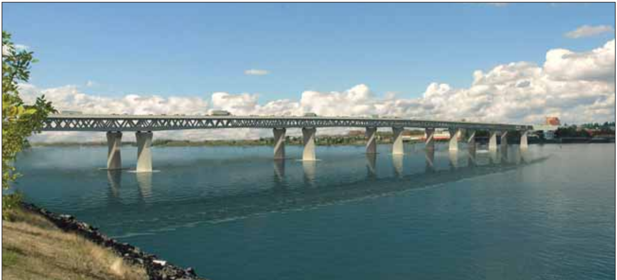
Exhibit 2.2-3 Composite Deck Truss Bridge Type
