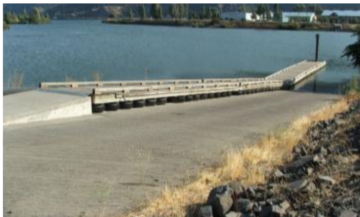
Figure A-17. Port of Klickitat Bingen Point Industrial Park
