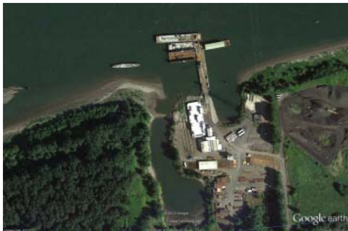
Figure A-22. Sundial Marine Tug & Barge Works
