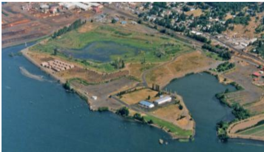
Figure A-16. Port of Klickitat Bingen Point Industrial Park
