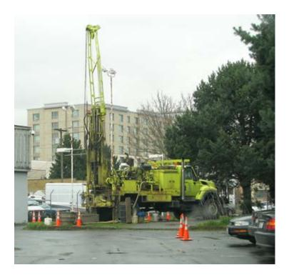
Geotechnical investigations will obtain more information about the physical properties of soil and rock, such as stability and drainage rates. Field crews will obtain subsurface soil and rock samples through geotechnical borings, which are holes that are drilled into the ground. Approximately 35 borings measuring four inches in diameter will be drilled 30 feet deep. Holes will then be backfilled and repaved before crews move to a new location.
