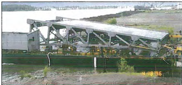
Bridge Fabrication—1 st Avenue & Duwamish (1996)
