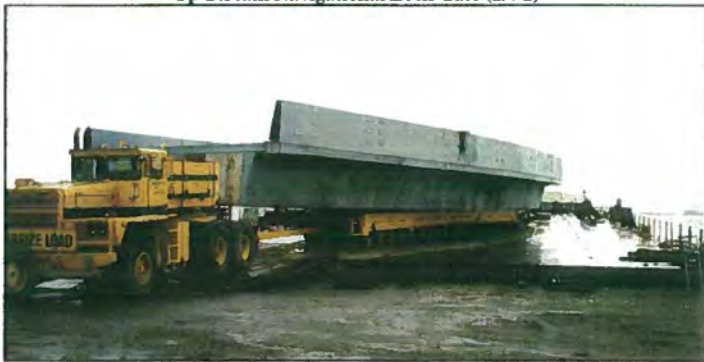
Orthotropic Tub Girder Fabrication—Nimitz Freeway (1995)
