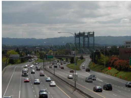
Exhibit 4-26. I-5 at Evergreen Road Overpass: Southwest at I-5 Bridge – View Point 11
