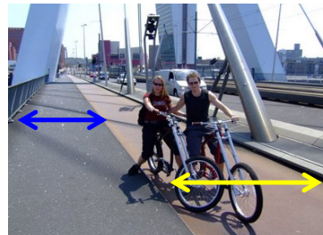
Erasmusbrug Rotterdam, Netherlands 6' sidewalks (2) 6' bike lanes (2) Total: 24'
