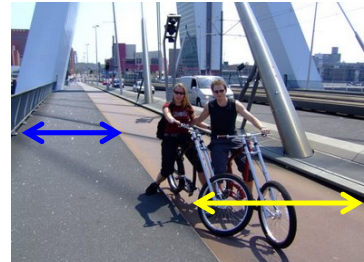
Eramusbrug Rotterdam, Netherlands 6' sidewalks (2) 6' bike lanes (2) Total: 24'
