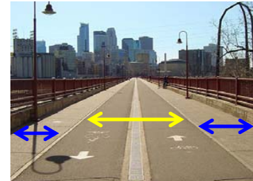
Stone Arch Bridge Minneapolis, MN Bi-directional bike path (1) Sidewalks (2) Total: 24'
