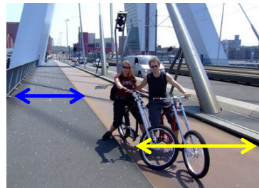
Eramusbrug Rotterdam, Netherlands 6' sidewalks (2) 6' bike lanes (2) Total: 24'
