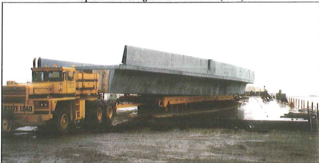
Orthotropic Tub Girder Fabrication—Nimitz Freeway (1995)
