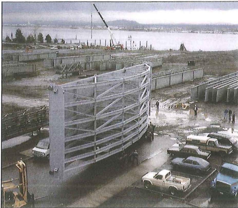
Up-Stream Navigational Lock Gate (1991)
