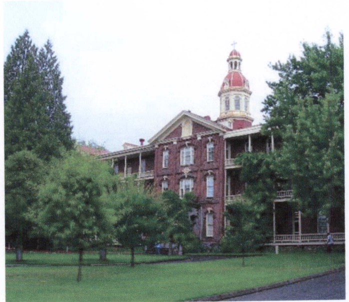
View of South facade
