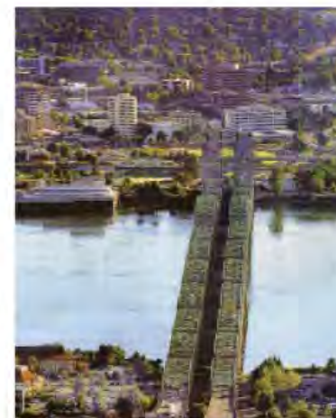
Existing Columbia River crossing
