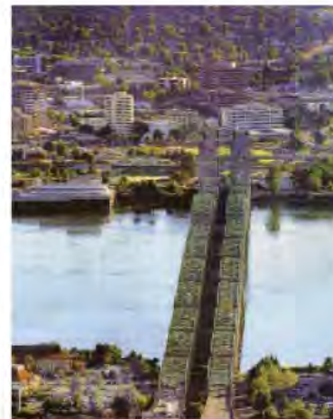
Existing Columbia River crossing
