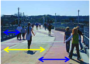
Pflugler Bridge Austin, TX 10' bi-directional bike path (1) 5' sidewalks (2) 15' observation deck Total: 20'
