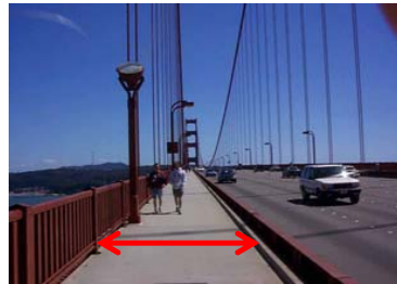
Golden Gate Bridge San Francisco, CA 10' shared-use path (1 full-time) 10' (5' clear) bike path (weekend) 1' raised above roadway Total 10' (15' weekend)
