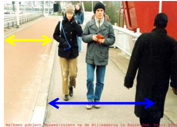
Willemsbrug Rotterdam, Netherlands 6' sidewalks (2) 6' bike lanes (2) Total: 24'
