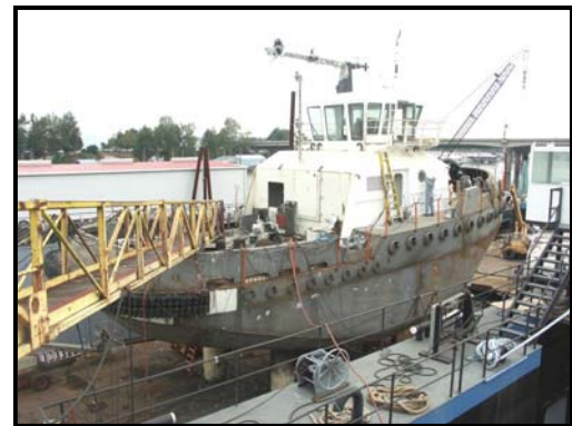
Showing construction of 80' 3800 hp tug in 2004
