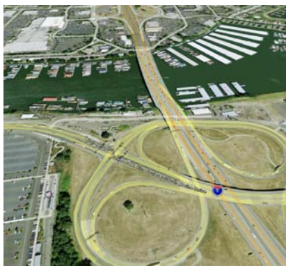
Existing I-5/Marine Drive Interchange
