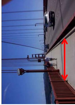
Golden Gate Bridge San Francisco, CA 10' shared-use path (1 full-time) 10' (5' clear) bike path (weekend) 1' raised above roadway Total 10' (15' weekend)
