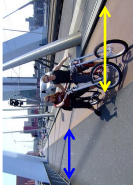
Eramusbrug Rotterdam, Netherlands 6' sidewalks (2) 6' bike lanes (2) Total: 24'
