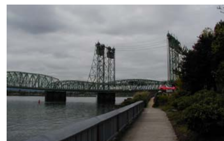
Exhibit 3.9-5 Bridges from Waterfront Park
