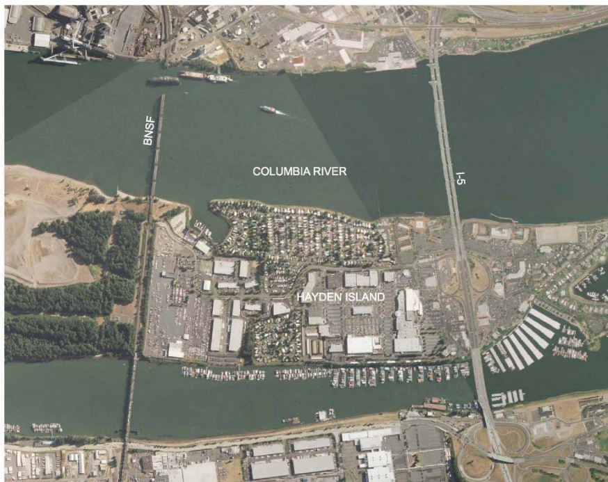
Exhibit 3.2-1 I-5 and BNSF Railroad Bridges
