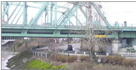
Exhibit 3.7-8 Existing Low Clearance at Waterfront Park
