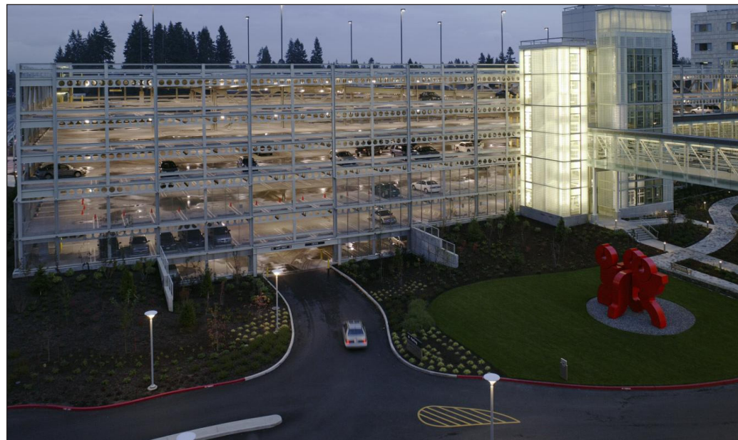
Legacy Hospital Parking Garage, Portland, Oregon
