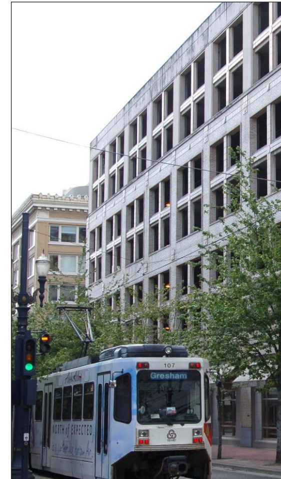
Pioneer Place Garage, Portland, Oregon
