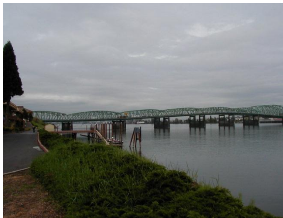
Exhibit 3-12. Hayden Island: Northwest looking at I-5 Bridge and Vancouver – Viewpoint 19
