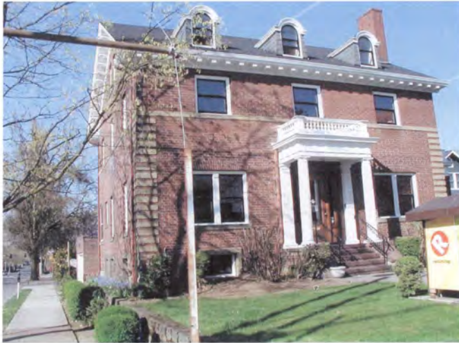
110 West 13 th Street Foster Hidden House
