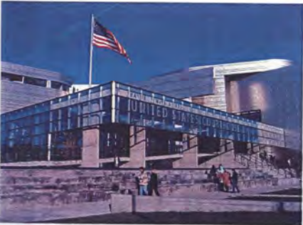
The two projects used as a process prototypes leading to the Program Guide:
