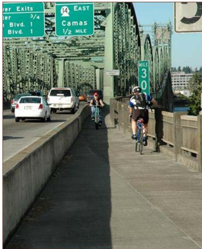
Figure 3-17. Photograph of Existing Non-Standard Multi-Use Pathway
