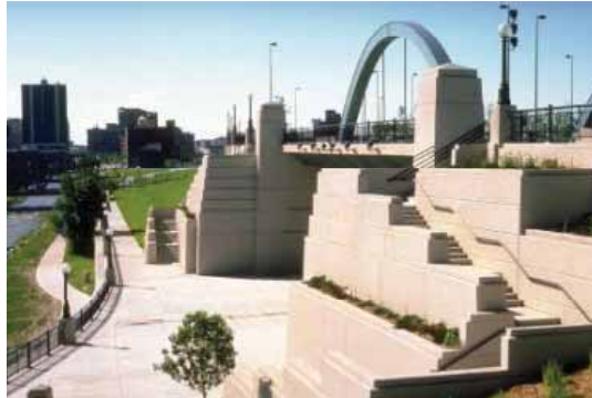
An example of a station that creates a gateway and sense of arrival (Source: ZGF)
