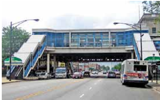
An example of an elevated station that is accessible from both sides of the street, provides transparency, and protects riders from the rain and wind (Source: ZGF)
