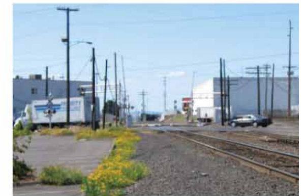
8th Street crossing BNSF Rail lines
