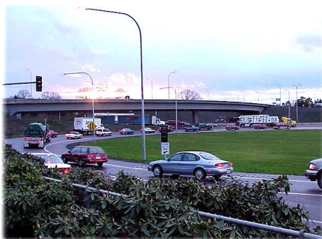
Southbound on-ramp to I-5 at SR 14
