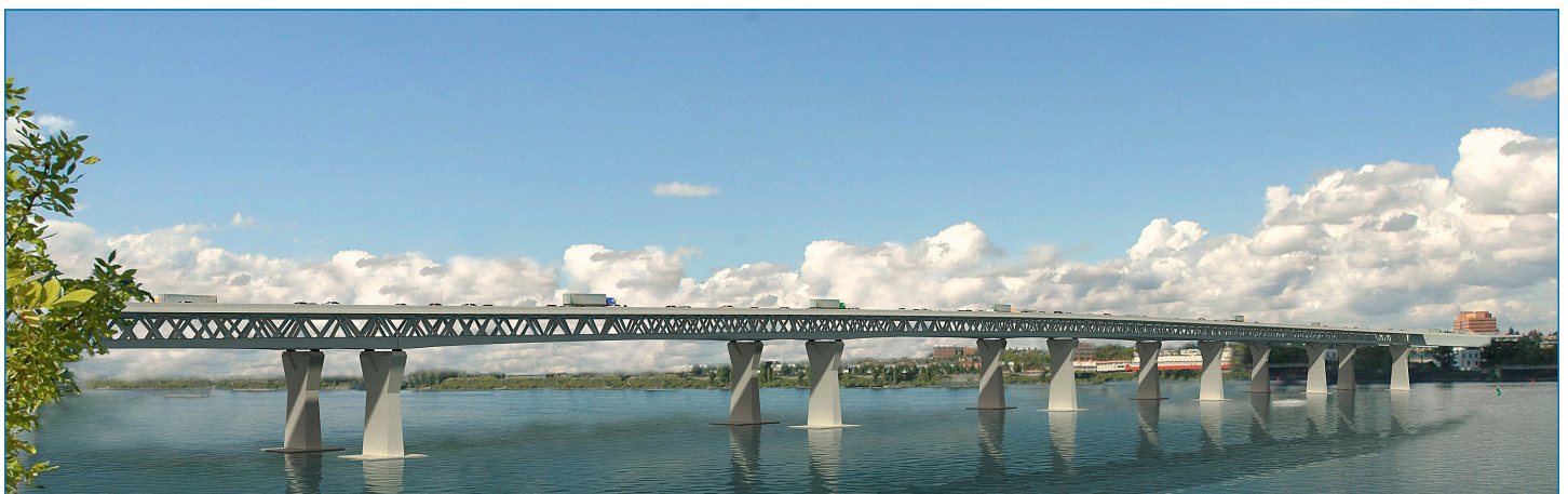
Concept rendering of deck truss bridge for replacement I-5 bridge. Architectural designs have not been completed.
