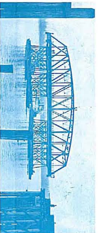
Bridge span is floated into place by barge during construction of the 1917 Interstate Bridge Oregon Historical Society, OHS 101203
