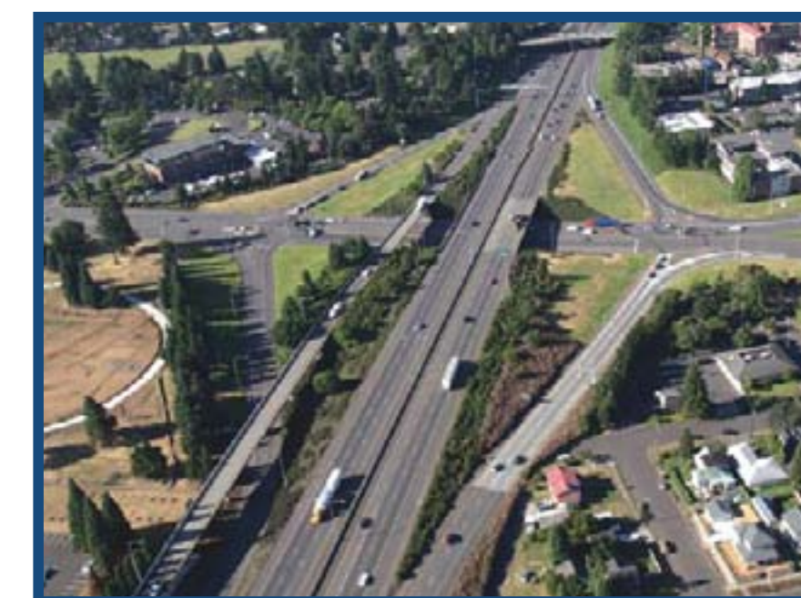
Mill Plain I-5 southbound
