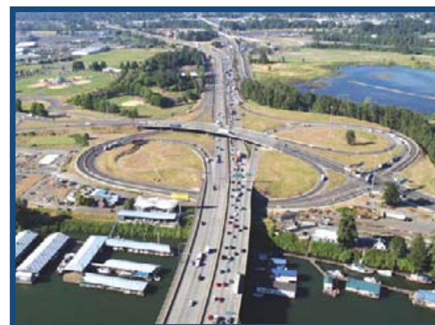
Marine Drive I-5 southbound
