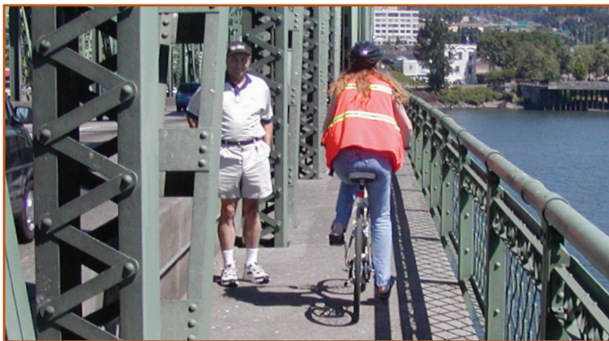
Today's Interstate Bridge paths are too narrow for pedestrians and bicyclists to safely pass each other.
