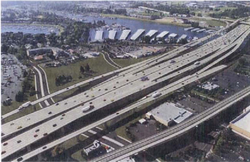
Columbia River Crossing conceptual drawing, looking south, showing the new bridge with light rail access along the west (lower right in drawing) side.
