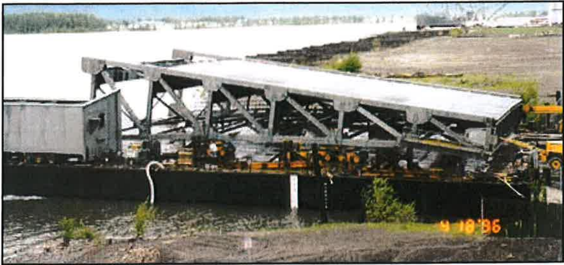
Bridge Fabrication—1 st Avenue & Duwamish (1996)
