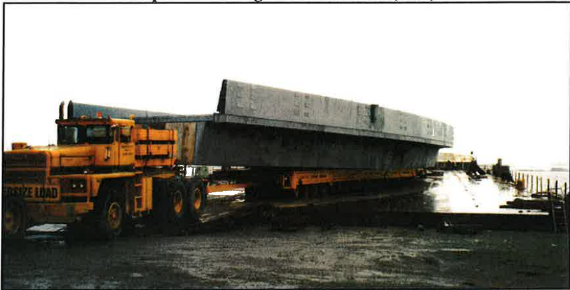
Orthotropic Tub Girder Fabrication—Nimitz Freeway (1995)
