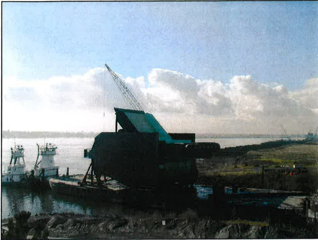
950 Ton Removable Spillway Weir for Ice Harbor Lock and Dam (2005)
