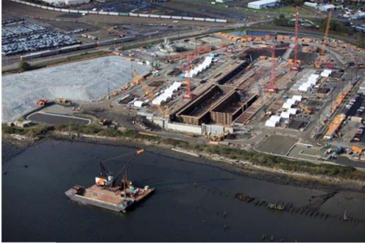
FIGURE 1-2. ABERDEEN CASTING BASIN UNDER CONSTRUCTION
