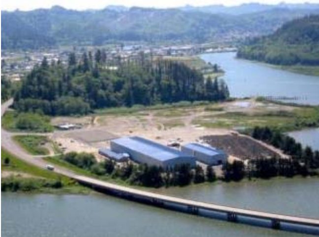
FIGURE 1-3. AMERICAN BRIDGE, REEDSPORT
