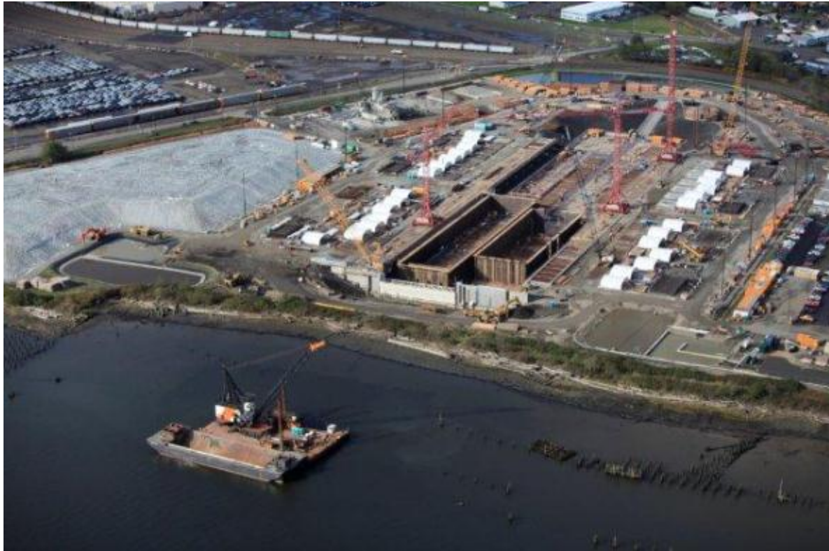
FIGURE 3-3. SR 520 PONTOON CONSTRUCTION SITE (ABERDEEN)
