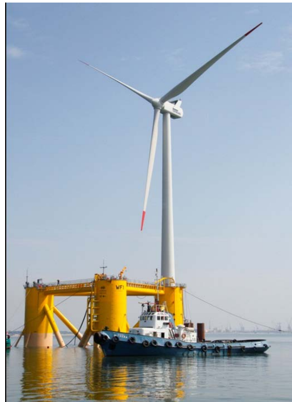
Figure 2. 2.0 MW Prototype Offshore Wind Turbine on Semi-Submersible
