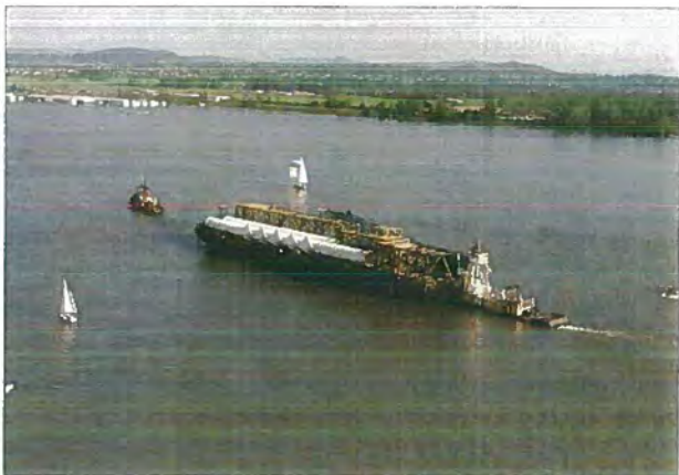
Georgia Pacific (Toledo, Oregon)—1,680 Foot Wood Chip Material Handling System (1975)
