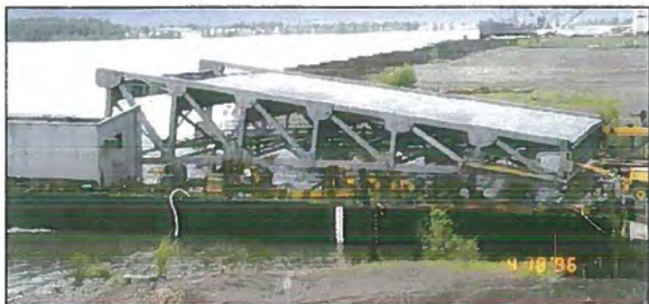
Bridge Fabrication—1 st Avenue & Duwamish (1996)
