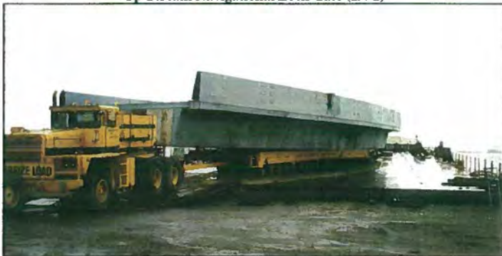
Orthotropic Tub Girder Fabrication—Nimitz Freeway (1995)
