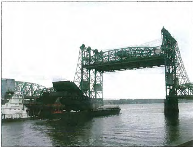
1,000 Ton Removable Spillway Weir for Lower Granite Dam (2001)
