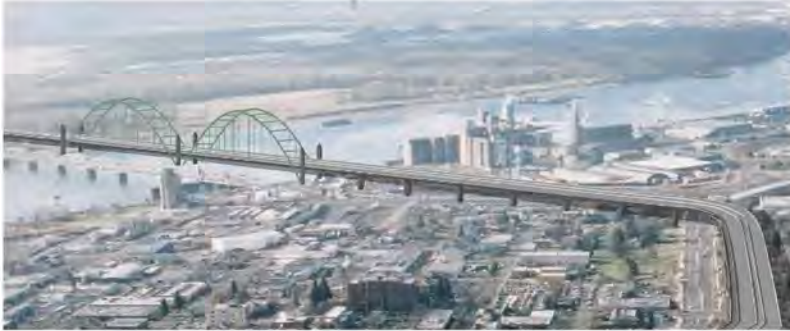
-Thirdbridgenow.com – Northern Bridge-
