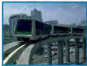
People Mover/ Automated Guideway Transit
