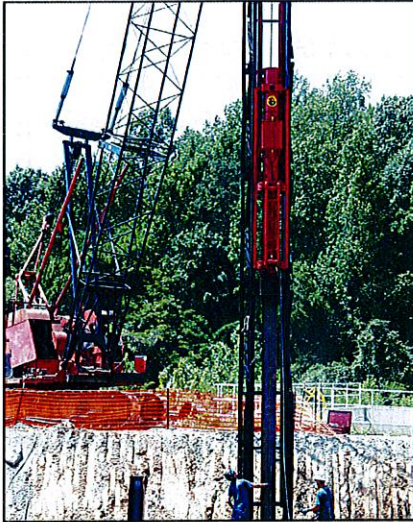
D19-42 driving H-beam.
