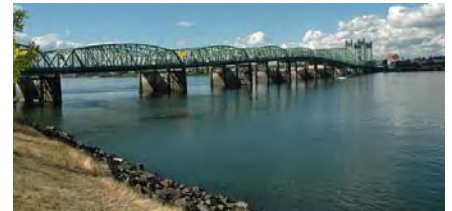
Exhibit 3.14-3 Columbia River Main Channel and I-5 Bridges
