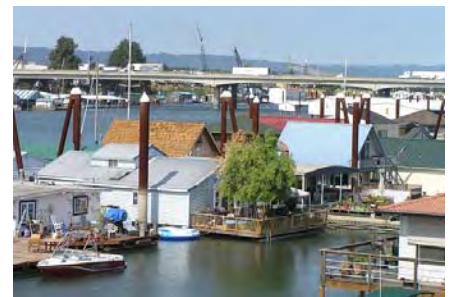
Exhibit 3.14-4 North Portland Harbor Channel and I-5
