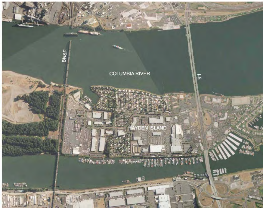
Exhibit 3.2-1 I-5 and BNSF Railroad Bridges
