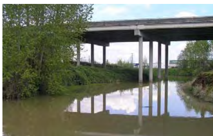
Exhibit 3.14-2 I-5 Crossing the Columbia Slough
