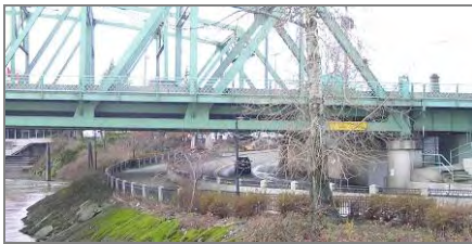
Exhibit 3.7-8 Existing Low Clearance at Waterfront Park
